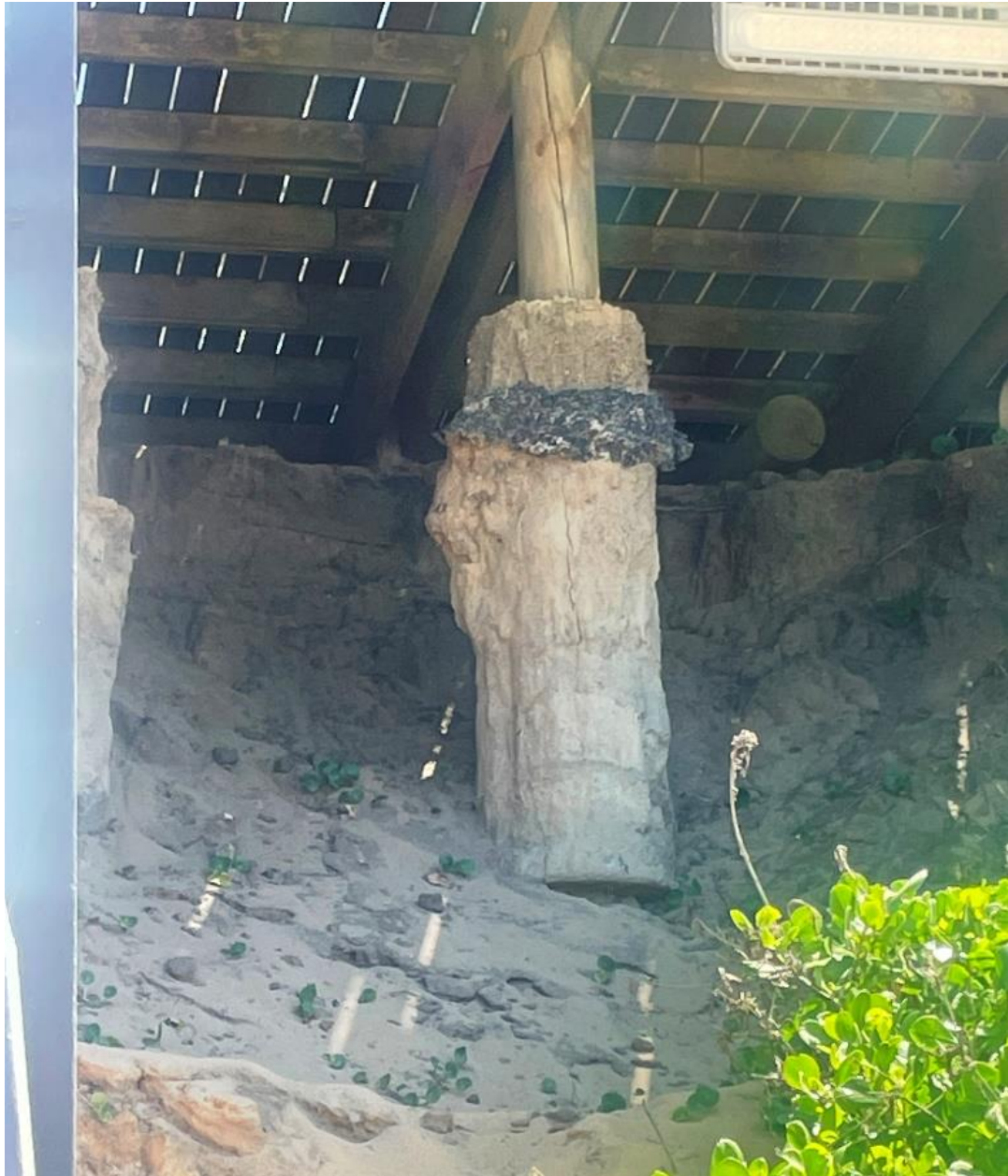
P12: Undermined pier at No 47 Ocean View Drive
