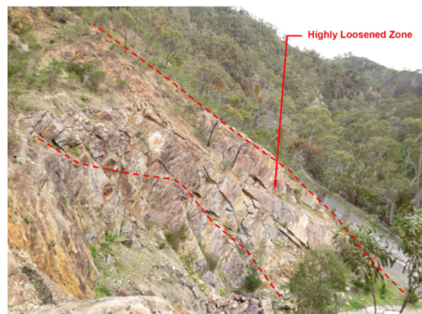
Fig. 6. Kangaroo Creek Dam site showing persistent valley stress relief sheet joints parallel to ground surface and resulting loosening of the rock with open joints. The sheet joints cross-foliation and tectonic joints within the schist and gneiss. Photograph courtesy of GHD and SA Water.
