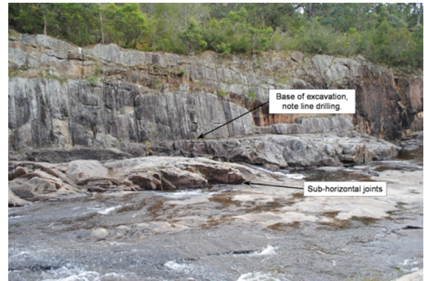
Fig. 9. Brogo Dam spillway showing erosion controlled by persistent sub-horizontal joints.
