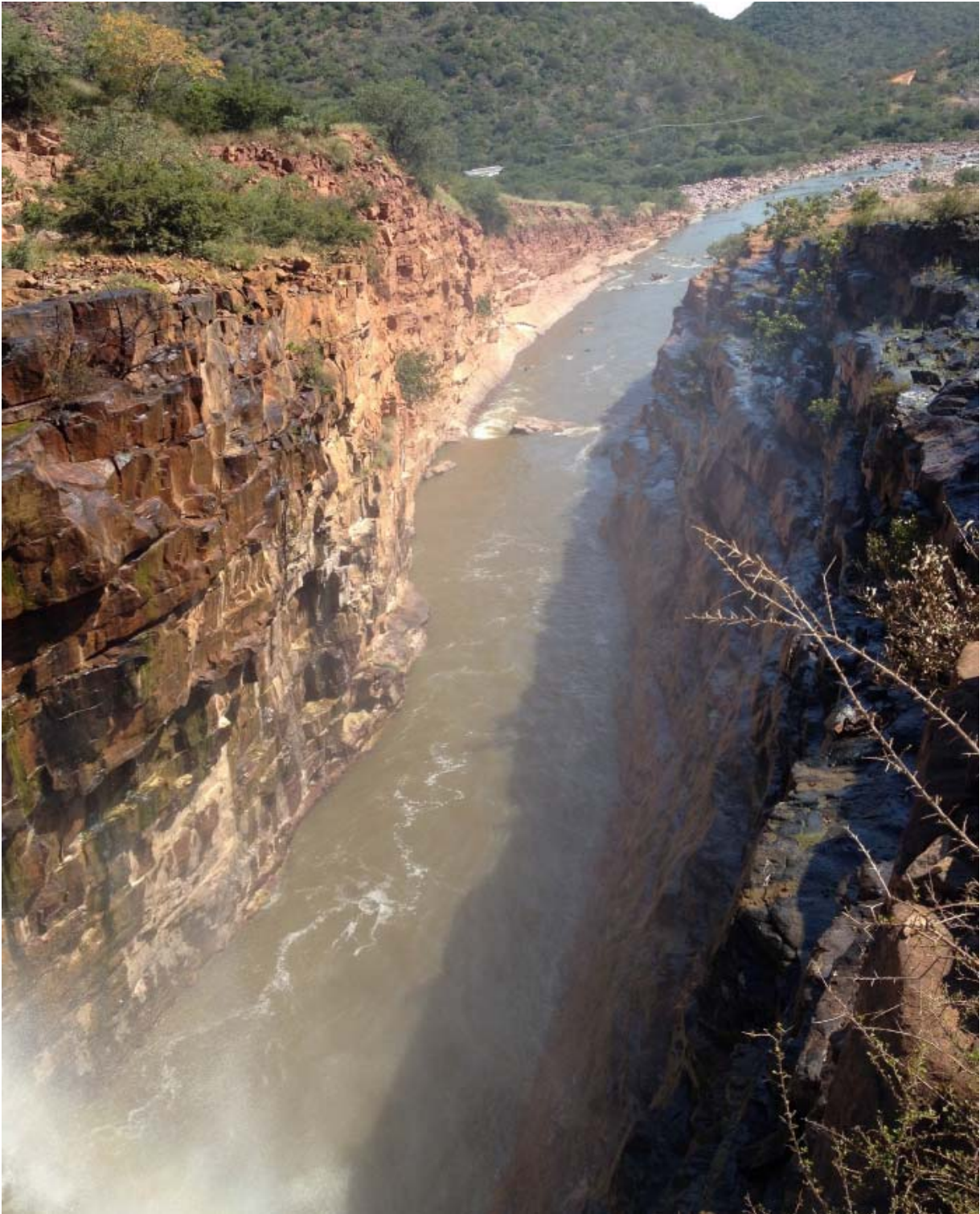
Figure 44 – View of the large erosion channel at Mokolo Dam (South Africa, photo SE Pells)
