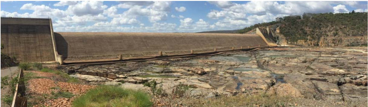
Figure 14 – Overview of Burdekin Falls Dam
