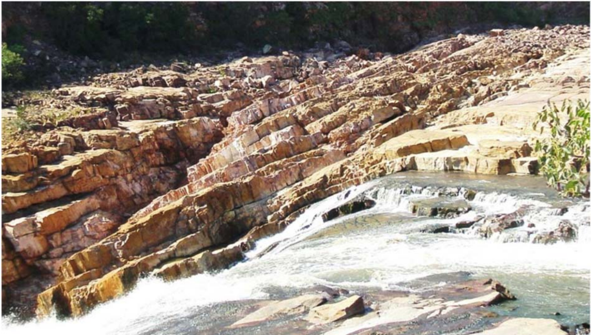
Figure 12 – Down-dragged beds adjacent to the thrust fault that passes through the spillway at Mokolo Dam
