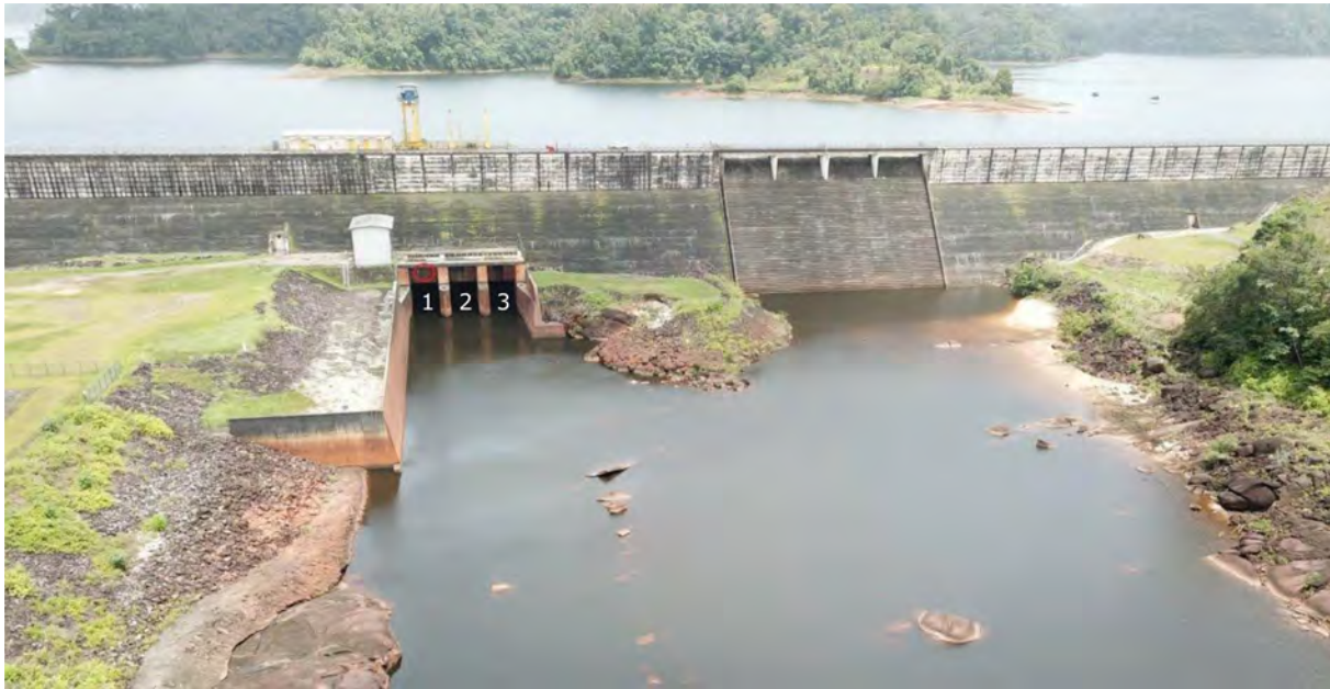
Figure 4: View of bottom outlet (showing numbering convention) and overflow spillway (1 July 1995)
