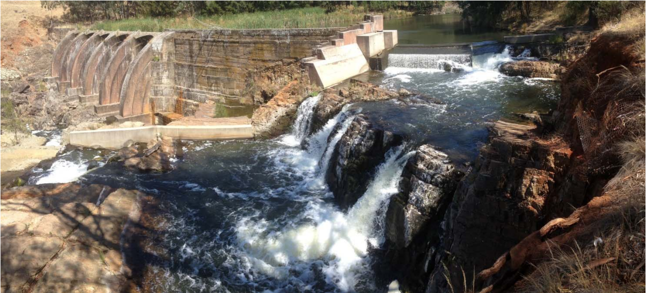
Figure 12 – Junction Reefs dam spillway, January 2014
