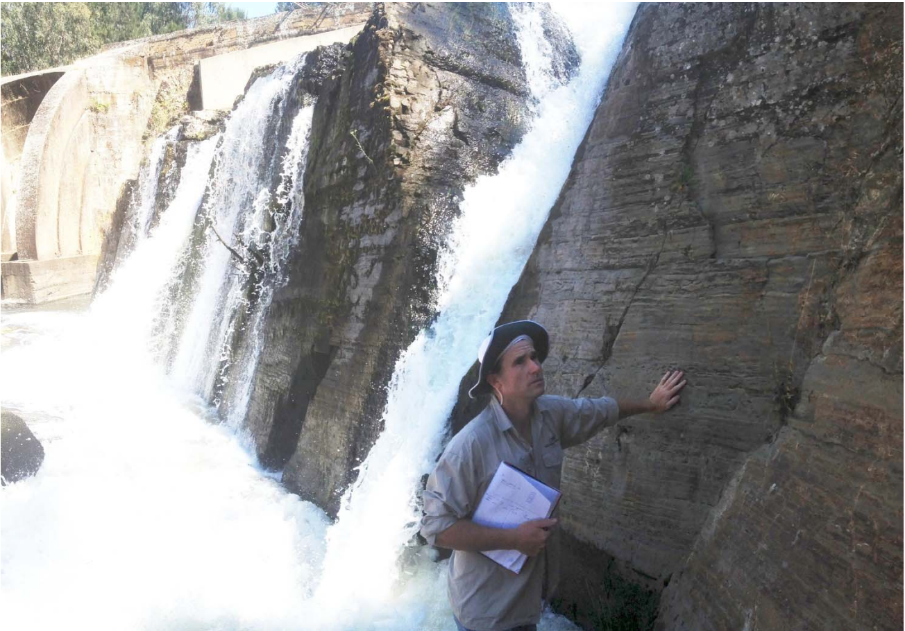
Figure 13 – First cascade of Junction Reefs dam spillway, January 2014
