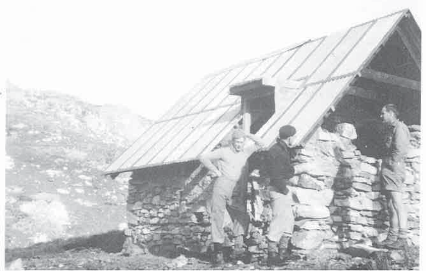
Below: Roof on, but sidewalls incomplete - probably April or May 1938
