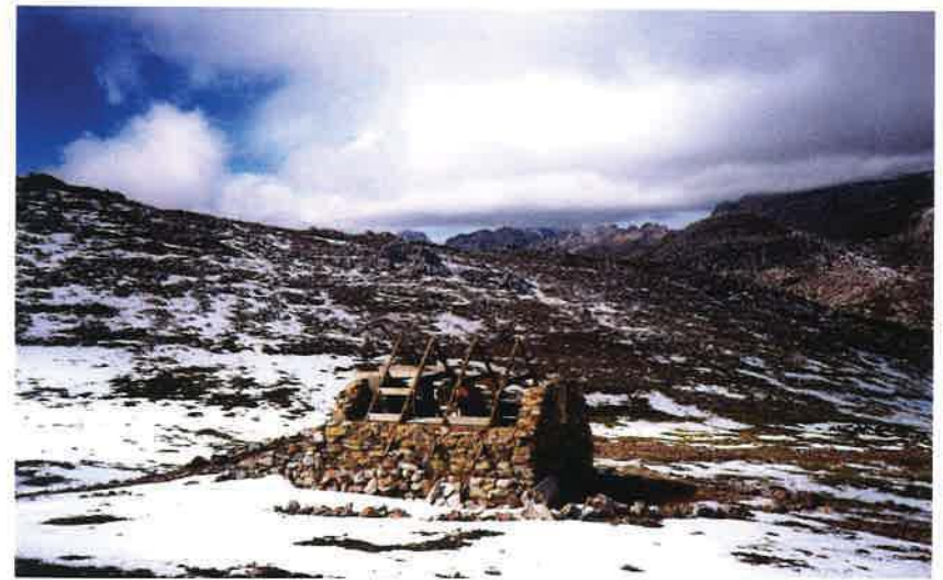
Below: The damaged hut after the storm
