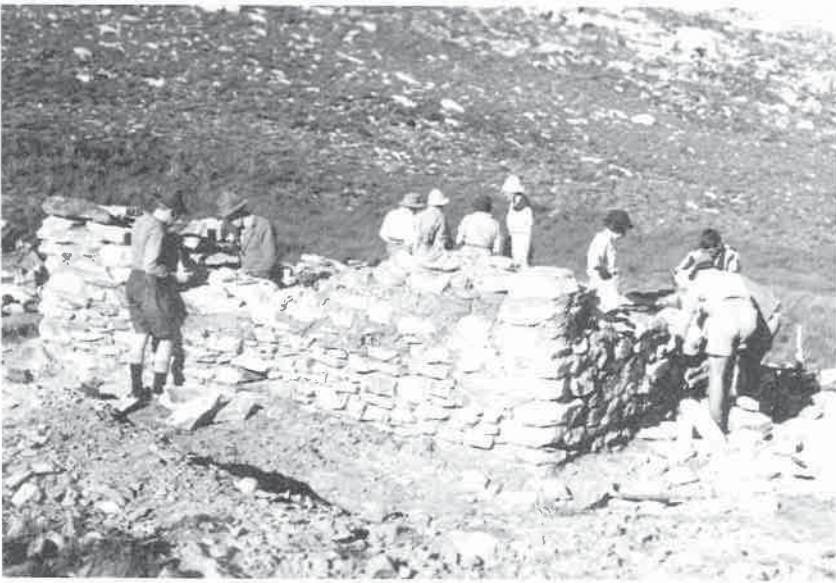
Below: Work on the wall - probably May 1937
