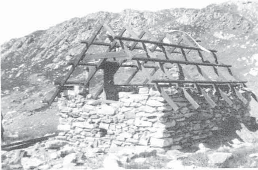
Above: Roof frame completed - February 1938
