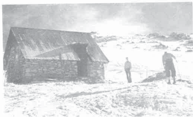
Below: The hut with sidewalls not completed - probably winter of 1937
