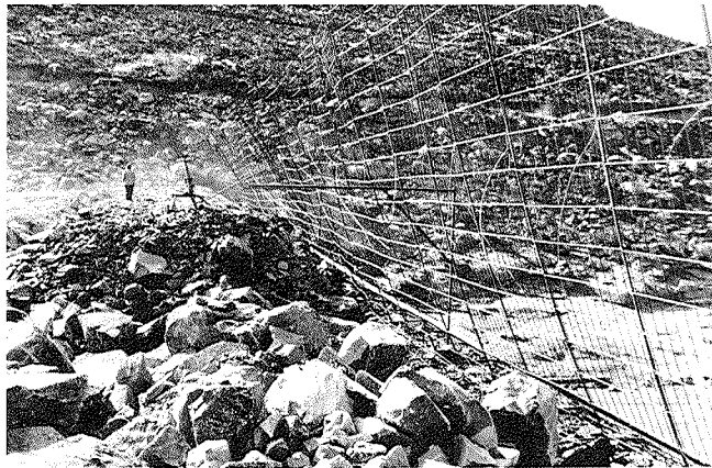
FIG. 7.—Rockfill Being Placed Behind Prefabricated Mesh Panels
